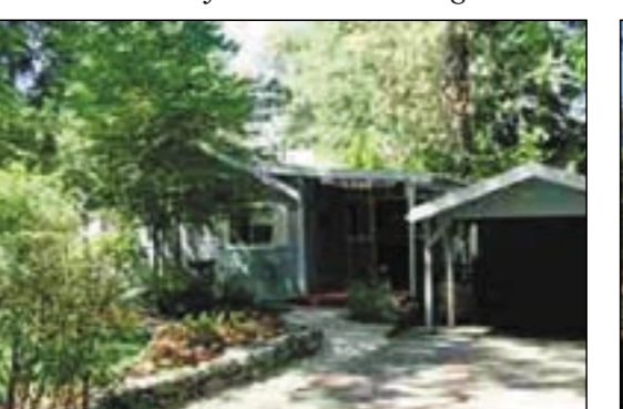
Vintage Miner's Cabin... 2bd/1ba; all useable parcel w/great yard & big trees; 1 block to Union Hill school; close to Empire Mine State Park; electrical, plumbing, redone in 1990; new roof in 2000. (MLS# 1027032) $324,500
