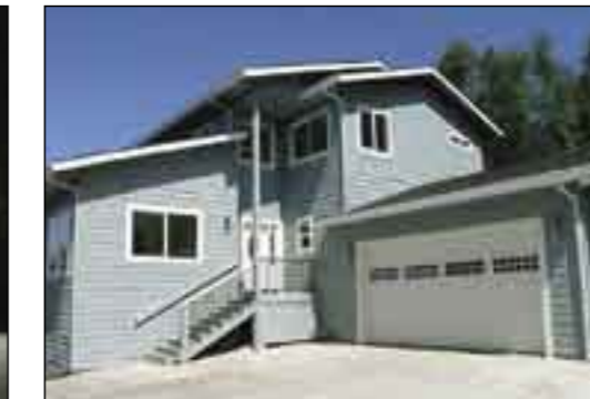
New Home Construction... 3bd/2.5ba; many custom features; great rm. floor plan + separate den & frml dng. rm.; great kitchen w/bkfst. nook. (MLS# 1026997) $649,500
