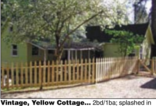
Vintage, Yellow Cottage... 2bd/1ba; splashed in a stream of sunshine amongst the tall cedars & pines of Peardale; charming; recently gone through and all inspections in file. (MLS# 1025050) $365,000
