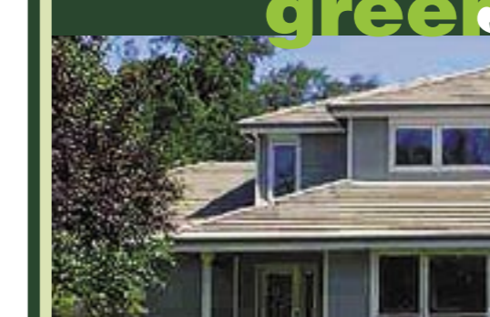
Green, Healthy & Natural... 3bd/2.5ba; live in style, luxury and comfort; advanced solar building architecture—1,560 watts, fully automatic, solar electric system, solar hot water and re-circulation system; 2x6 exterior walls with applied sound-proofing insulation; 40-year ceramic tile roofing; exterior European rolling window shutters; Energy Star appliances throughout; beautiful custom home with quality features throughout; great room floor plan with vaulted ceilings; open kitchen with solid granite counters, double ovens and island cook top; formal dining room just off the kitchen; private master suite with walk-in closets, double sinks in slab granite counters, jetted tub plus walk-in granite shower; two outdoor living areas with great views of the landscaped yard; 3-car garage plus additional parking areas. (MLS# 1025829) $549,950
