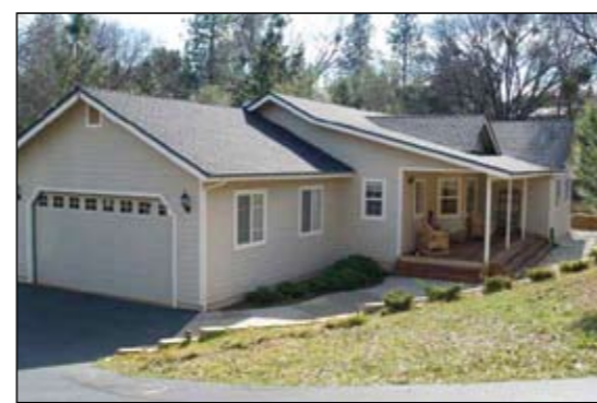
Newer, Light & Bright Home on 1 Acre... 3bd/2ba; in good commuter location; great rm. w/ vaulted ceiling leads to back deck w/spa overlooking lg. backyard; spacious ktchn. (MLS# 1028723) $419,000
